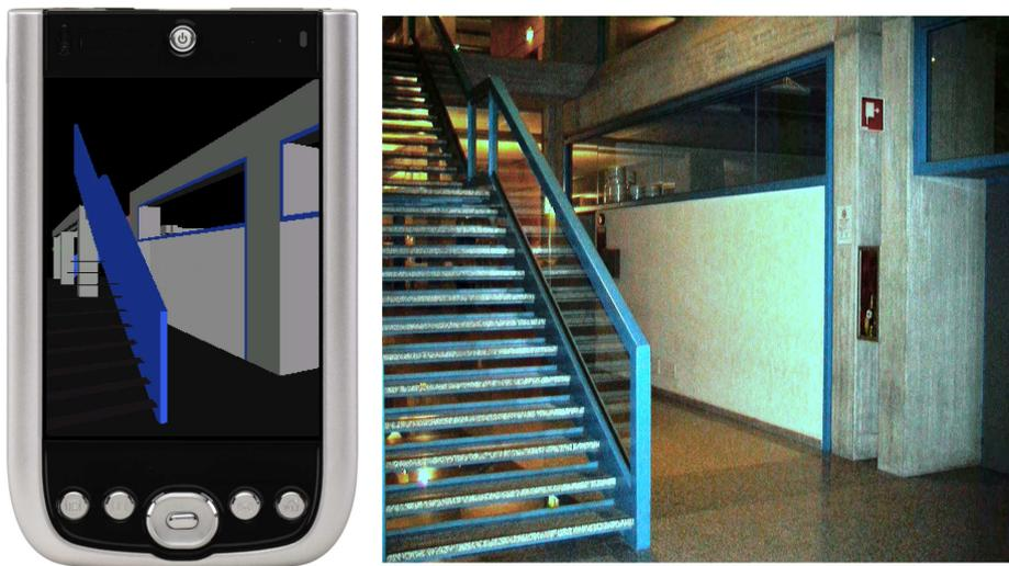
Figure 8: Part of the 3D model of the University of Udine (2 visible cells) with a photo of the corresponding area.
